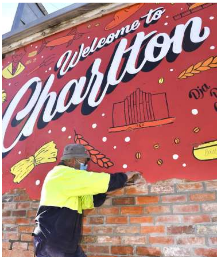
Above: Bricklayer, Rod Heritage, is pictured hard at work shoring up the building's exterior wall which houses one of Charlton's defining streetscape murals.
