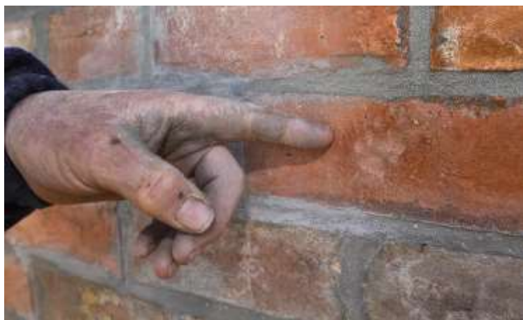
Above: The refurbishment of the Charlton Mensland western wall has revealed the added attraction of tiny possum feet imprints made more than a century ago.
