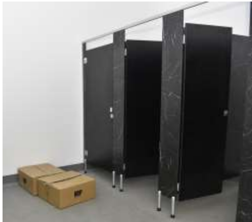
The cubicles in the women's toilets and the vanity basins are in the process of installation.
