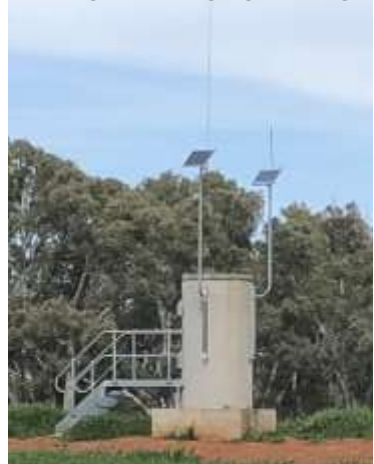
Yawong Weir new gauge housing.
