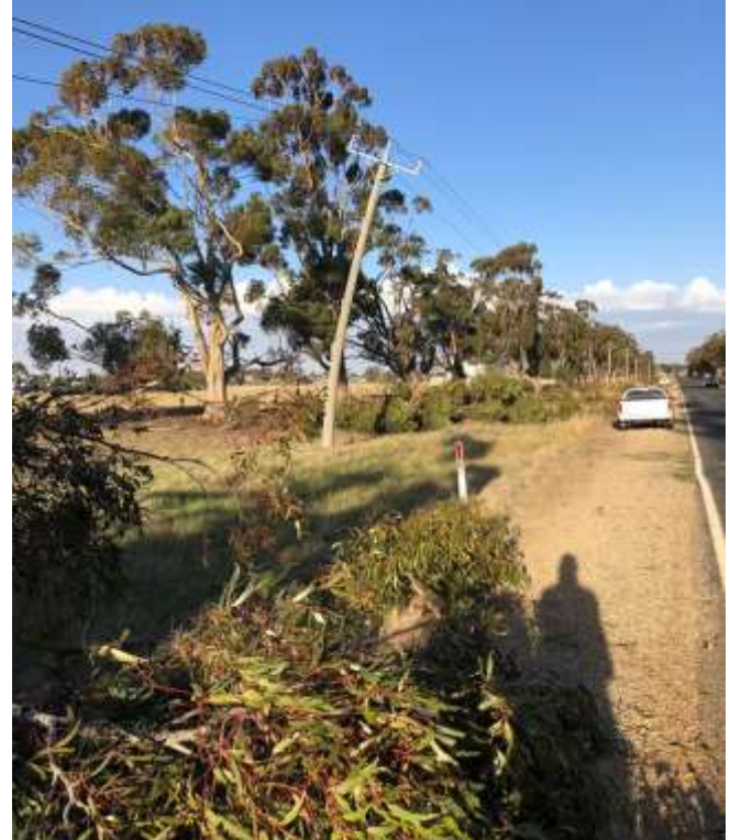
A cement power pole bent at an angle along the Borung Highway heading towards Donald.
