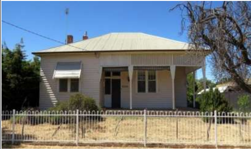
Homes like this do not come along very often, a renovator's dream. Three large bedrooms, high ceilings, huge yard and concreted, powered shed.
