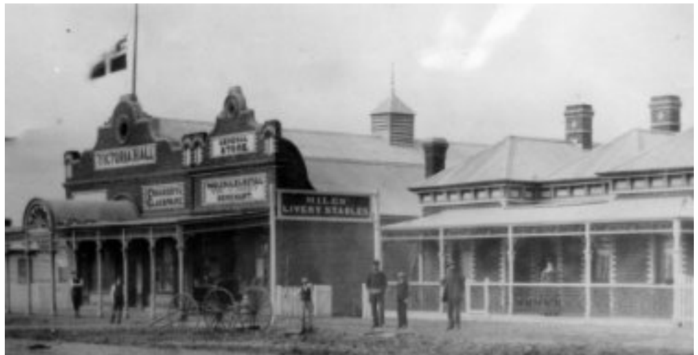
The Victoria Hall which was demolished to make way for the new hall.
